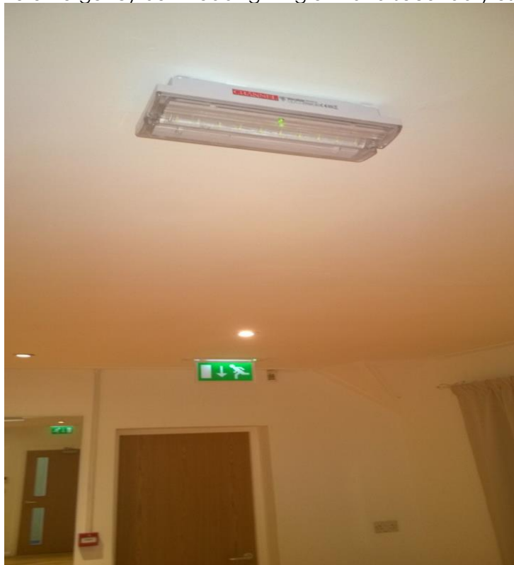
Fig 2. Fitness suite emergency bulk head lighting unit and secondary escape doorway
